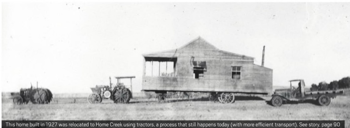
This home built in 1927 was relocated to Home Creek using tractors, a process that still happens today (with more efficient transport). See story, page 90
